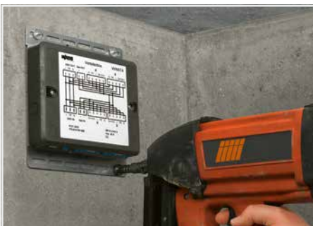
Securing the mounting plate with WINSTA® Box to the wall (e.g., via stud gun).
