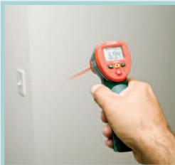
Check building for insufficient insulation
