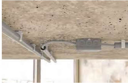
Fixing plastic insulating conduits
