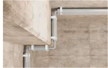
Fixing plastic insulating conduits
