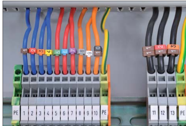
A secure way to clearly identify wires after they have been terminated.
