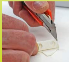
Fig. 7: Cutting the fit-up-aid „sail“ (D1) of the window frame bracket (D)
