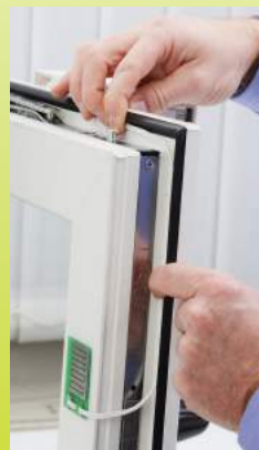
Fig. 31: Placing the cable sideways and fixing it with adhesive tape
