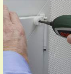
Fig. 16: Screwing the guide roller
