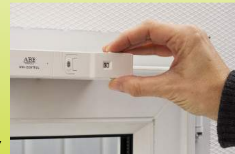
Fig. 33: Setting the time slice - clockwise
