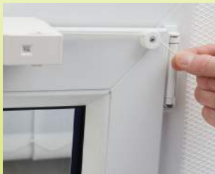
Fig. 17/18: Passing the release cord around the guide roller
