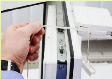
Fig. 23: Passing the cable outward
