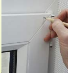
Fig. 14: Marking the position of holes for the guide roller
