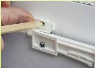
Fig. 5: Marking the position of screws for the window frame bracket
