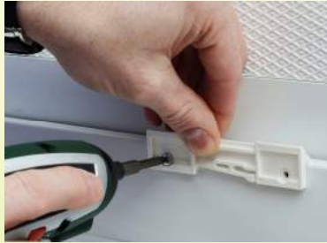
Fig. 3: Screwing on window casement
