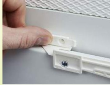
Fig. 4: Putting the window casement-bracket using the fit-up-aid (sail)
