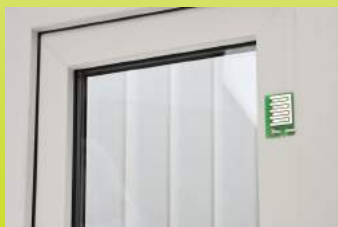
Fig. 32: Rain sensor completely fixed
