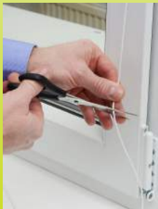
Fig. 19: Cutting the release cord into the desired length
