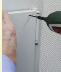
Fig. 15: Pre-drilling for mounting the guide roller
