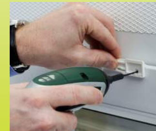
Fig. 2: Pre-drilling the holes at the window casement bracket (C)
