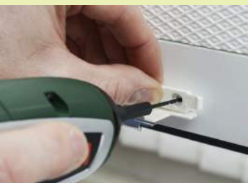
Fig. 6: Pre-drilling the holes at the window frame
