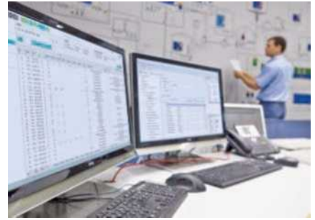
Remote control: Secure and continuous transmission of process data to the control center
