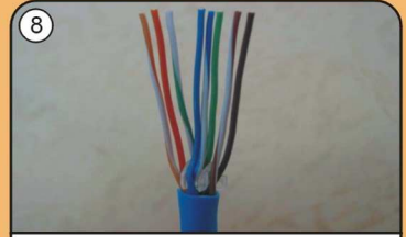
To Straighten the conductors
