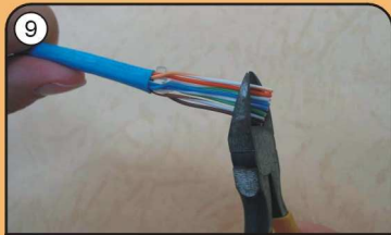
To cut off conductors neatly
