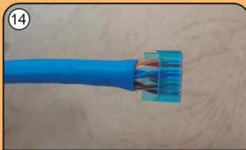
To see after cutting the conductors
