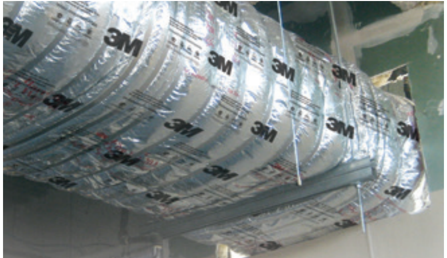
Flexible protection for grease and air ducts: 3M™ Fire Barrier Duct Wrap 615+ (pg 38)
