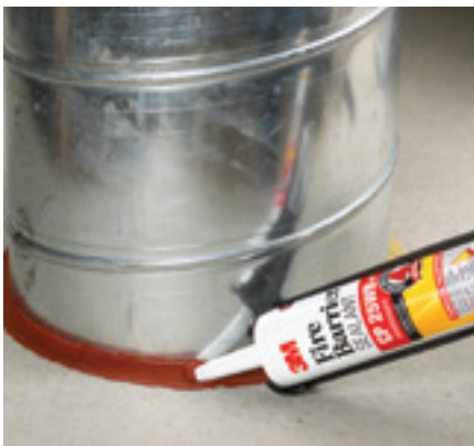
Sealing metal duct lines: 3M™ Fire Barrier Sealant CP 25WB+ (pg 32)
