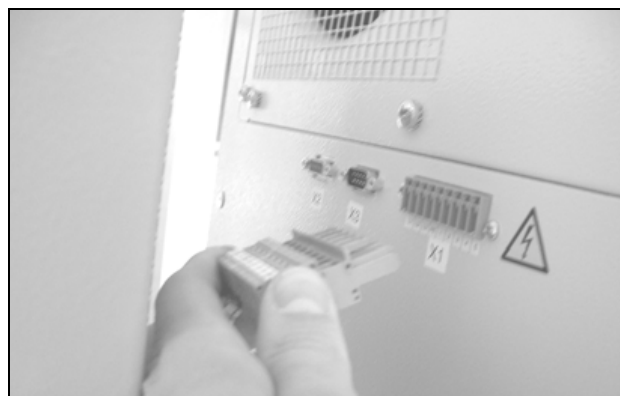
Fig. 34: Disconnect the mains plug
