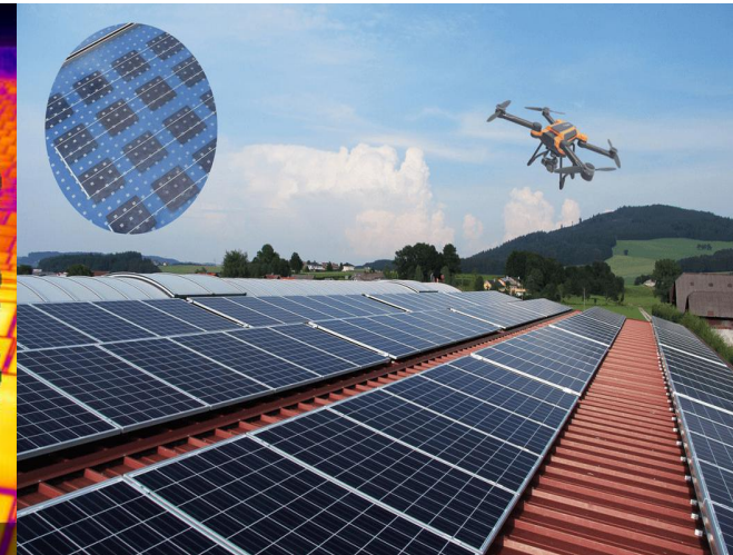
Inspect solar panel hot spots
