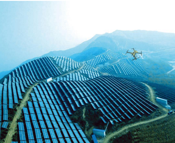
Solar power station inspection
