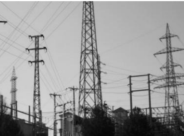
Power line inspection
