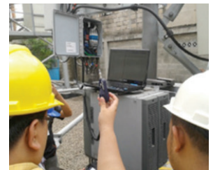
At the RRU (tower structure or rooftop)
