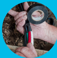
Wire and Cable Bundling
