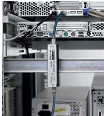
**Direct Grounding on the DIN Rail**
