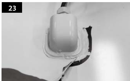
23 Remove friction tape .
