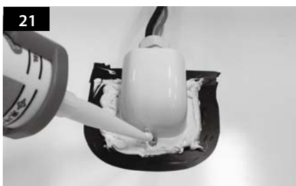
21 Apply silicone around and on the top of screws.
