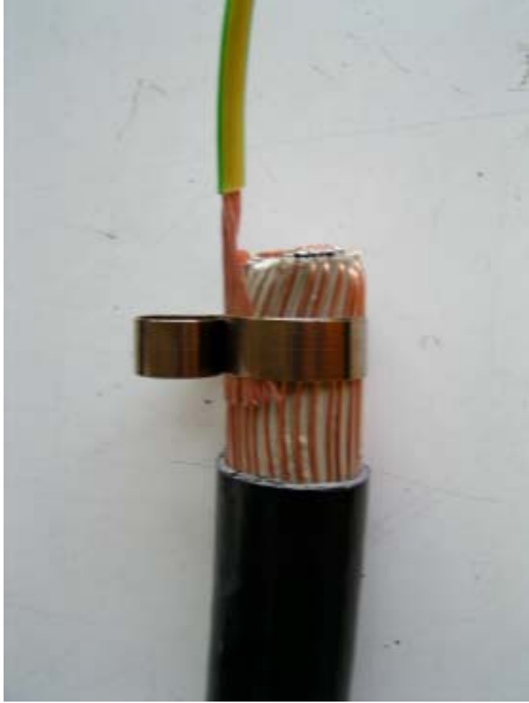
Fig. 1.3: Wrap the contact force spring SA KRF 50 V2A around both cables.
