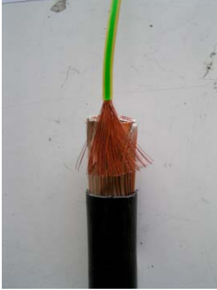
Fig. 1.2: Fan out the wires of the PE conductor and lay them on the shield.
