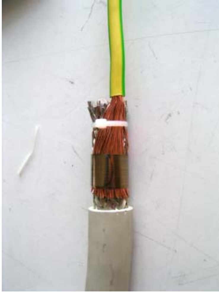
Fig. 3.3: Wrap the contact force spring SA KFR 22 V2A around both cables.
