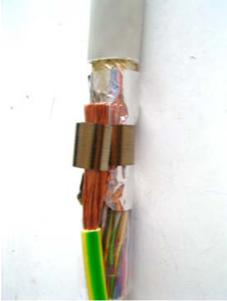
Fig. 4.3: Wrap the contact force spring SA KRF 22 V2A around both cables and ensure that the wires of the PE conductor are in contact with the sheath wire.
