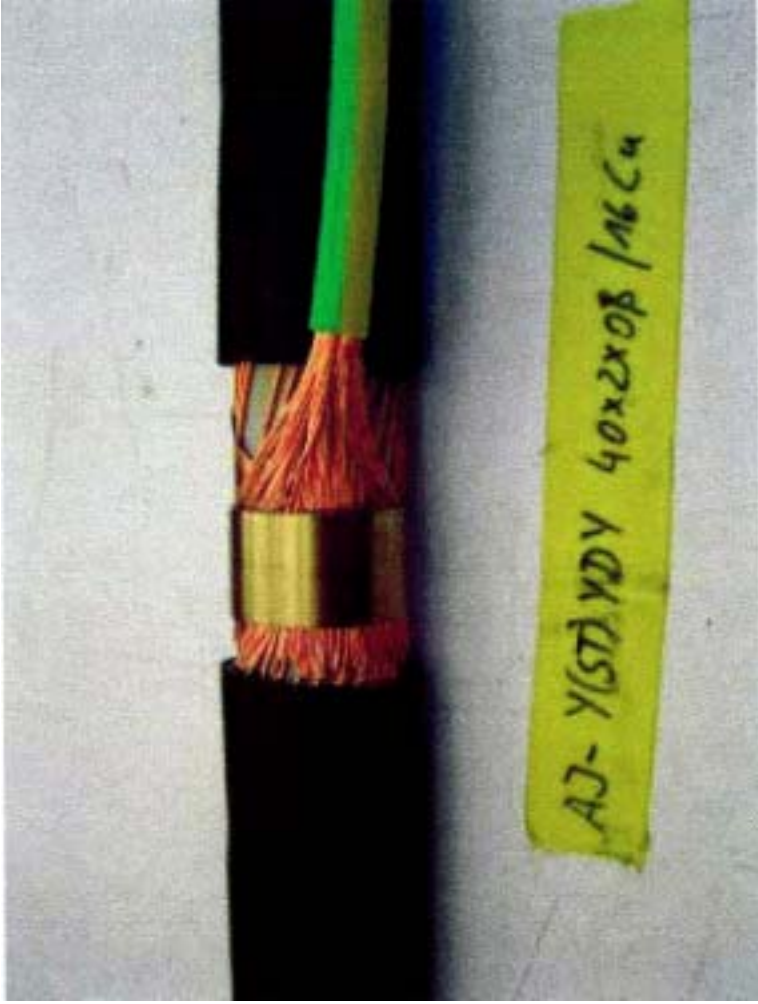
Fig. 2.3: Wrap the contact force spring SA KRF 29 V2A around both cables.
