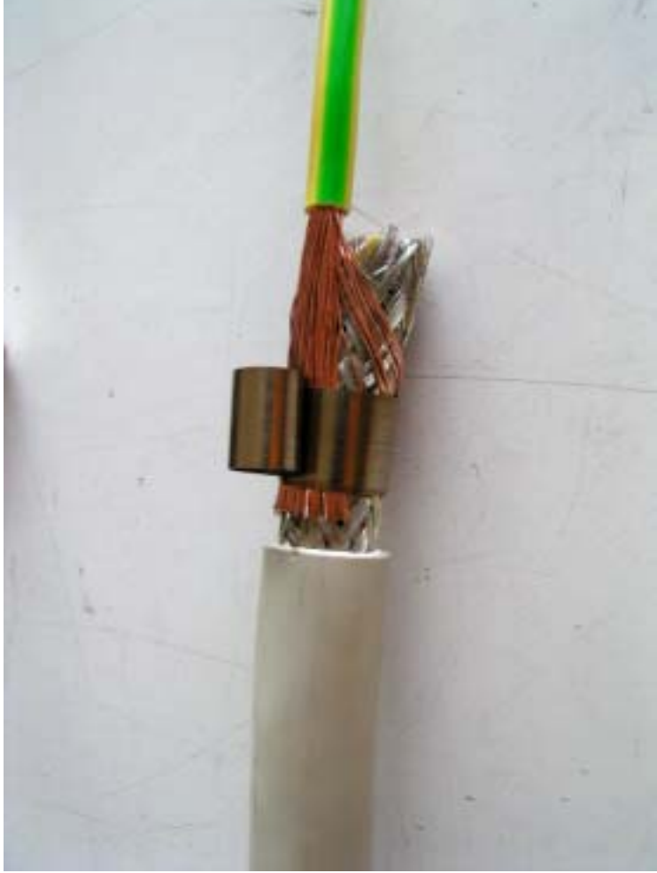
Fig. 3.3: Wrap the contact force spring SA KFR 22 V2A around both cables.
