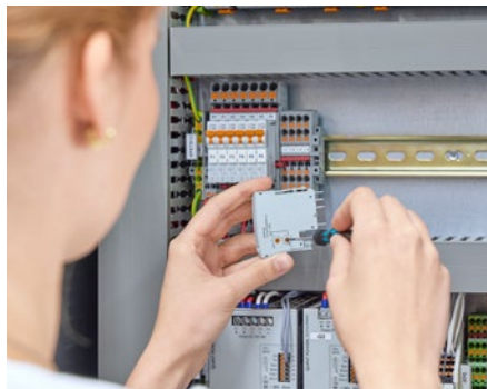
Easy configuration of the threshold value via rotary switch
